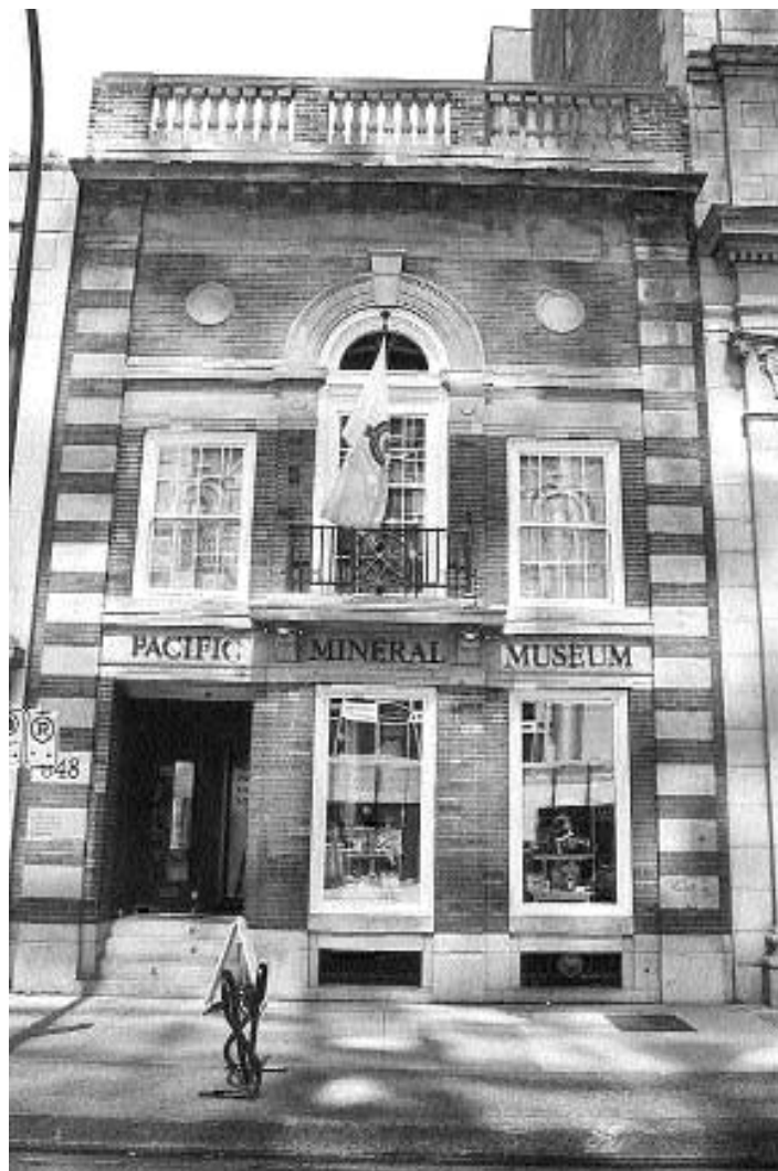
A new museum in a heritage building
